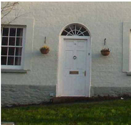
14 Typical Georgian 18th - early 19th century panelled door with fanlight above
