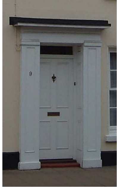
16 Typical Victorian 4 panelled door case
