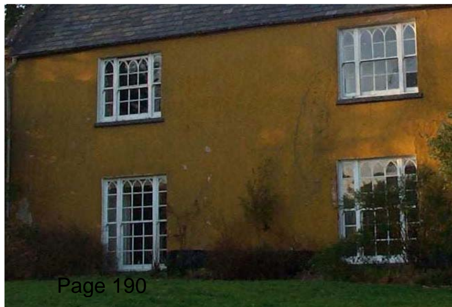
8 Vertical sliding sash with Gothic detail
