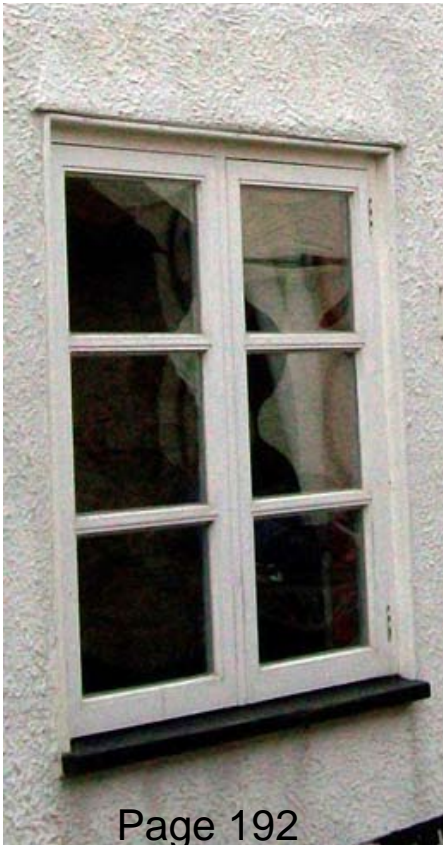
11 Flush fitting casement
