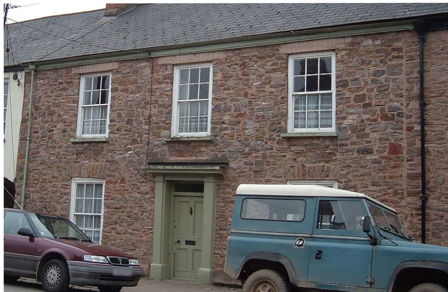
7 Vertical sliding sash
