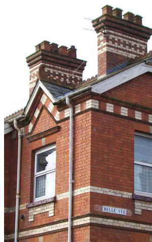
6 Distinctive chimney stack profile with attractive brick pattern and square chimney pots typical in Cullompton
