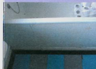
◀ Asbestos cement bath panels
