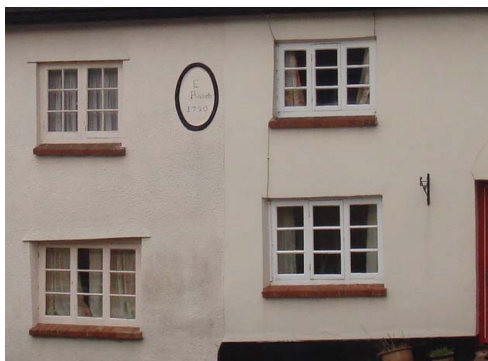
6 Side hung timber flush fitting balanced casement windows showing two typical glazing bar patterns
