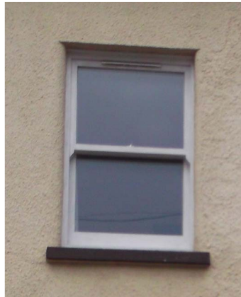
12 Vertical sliding sash
