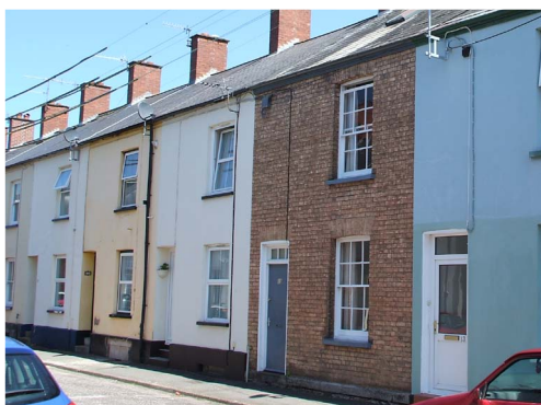
3 Terrace with an inappropriate mix of replacement windows and doors in contrast with one property retaining its original frontage design (including unpainted and unrendered brick)
